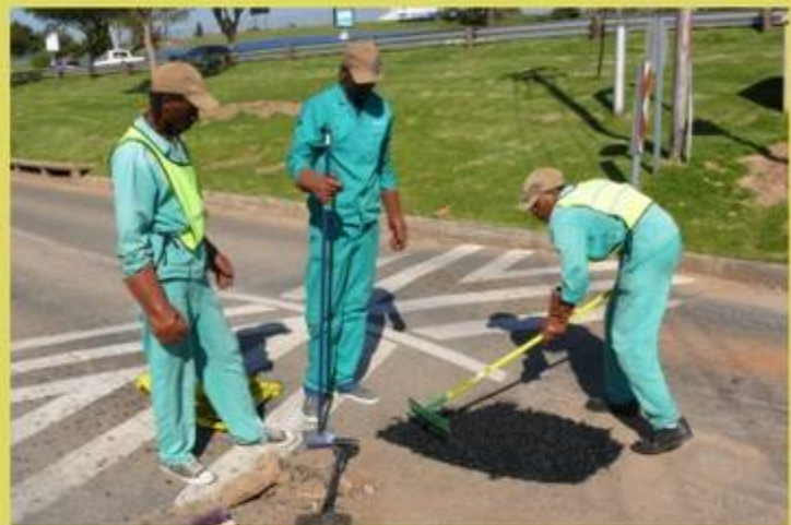
Pothole being fixed by the BECF team.
